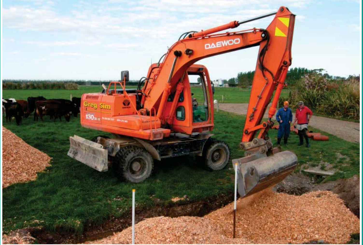
Bioreactor construction at a New Zealand dairy farm. Photo by Brandon C. Goeller.
