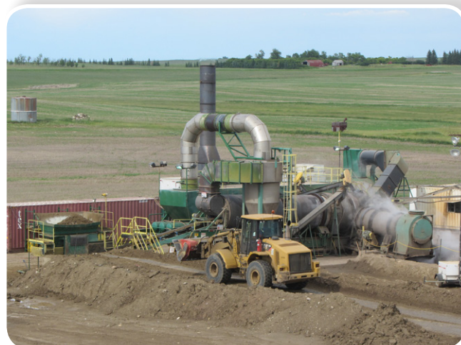
Thermal desorption unit used to treat the soils in this study.
